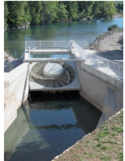
Bild 6: VLH-Turbine in Service-Position [1]
